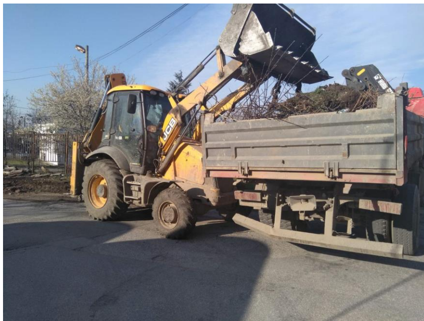
Fig. 7. Open dump rehabilitation in Karlovo, Bulgaria
